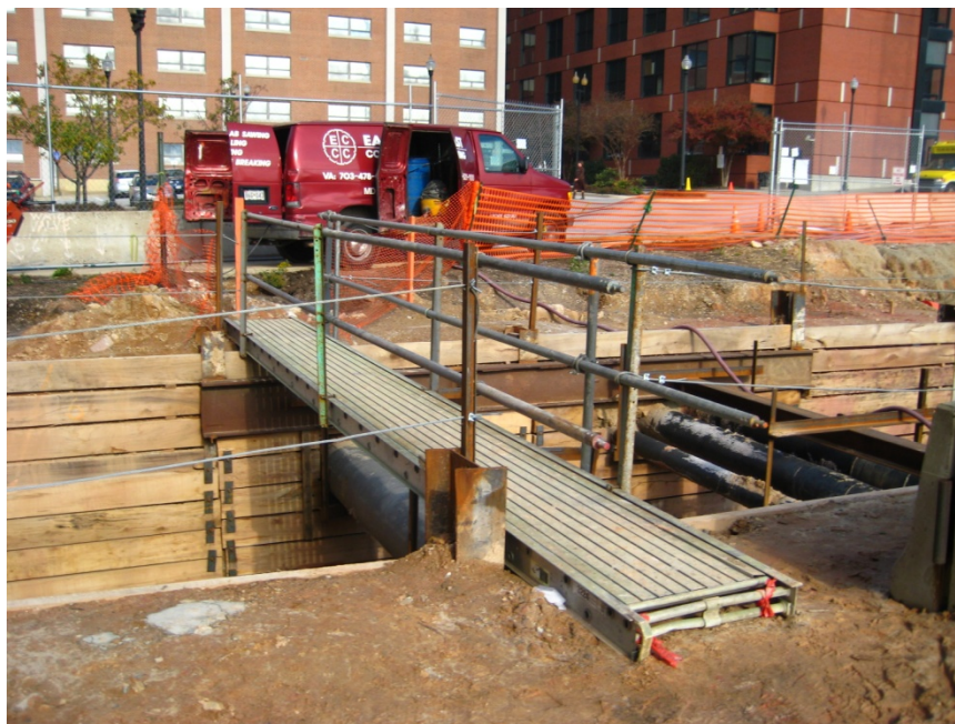
Temporary scaffold bridge over tunnel excavation
