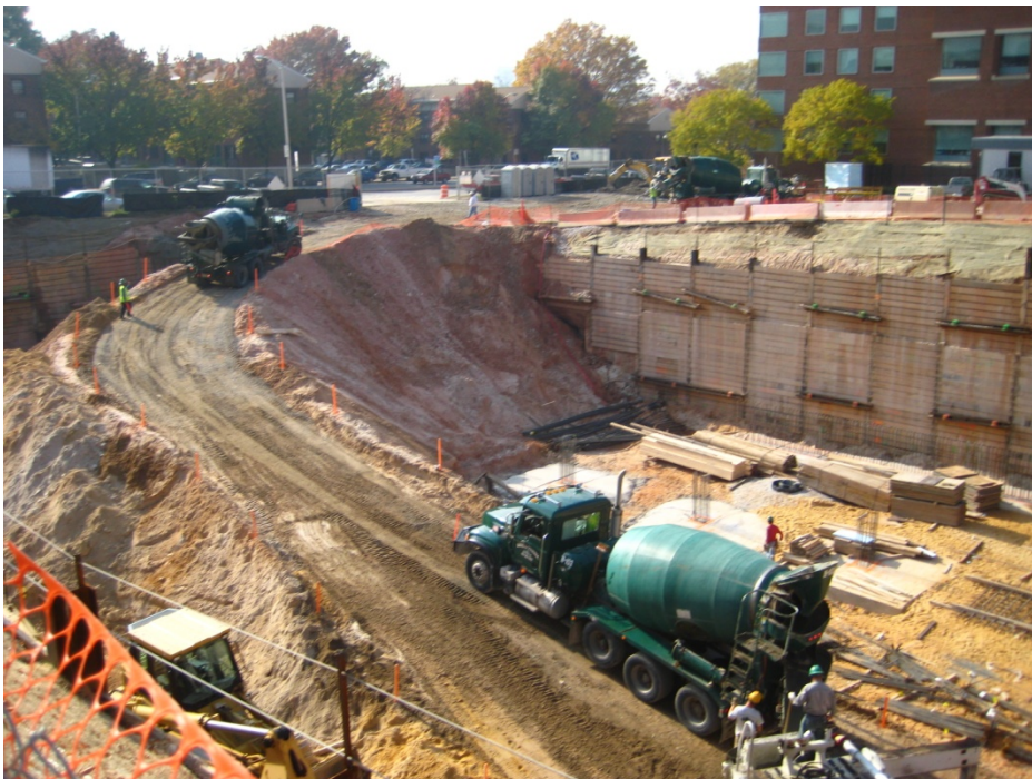
Temporary excavation ramp to be removed.
